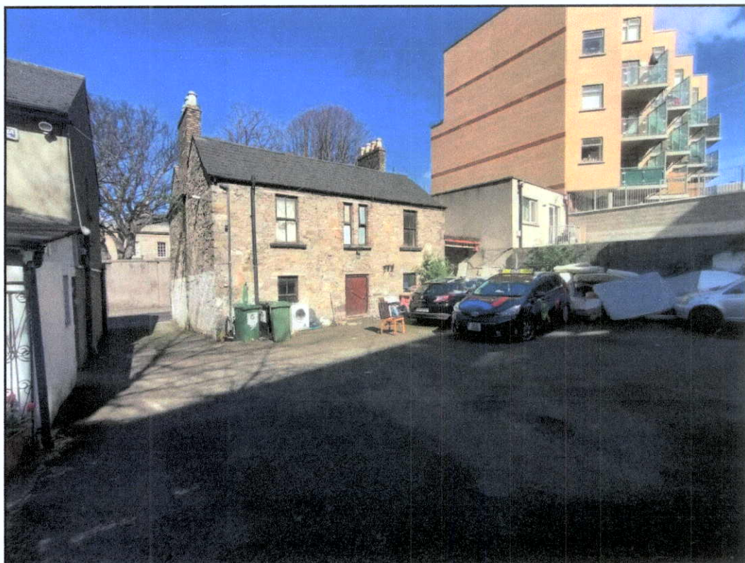
Plate 4 Rear yard, looking north-north-east.
